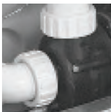
Vent air by slightly opening pump unions.
