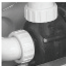
Vent air by slightly opening pump unions.
